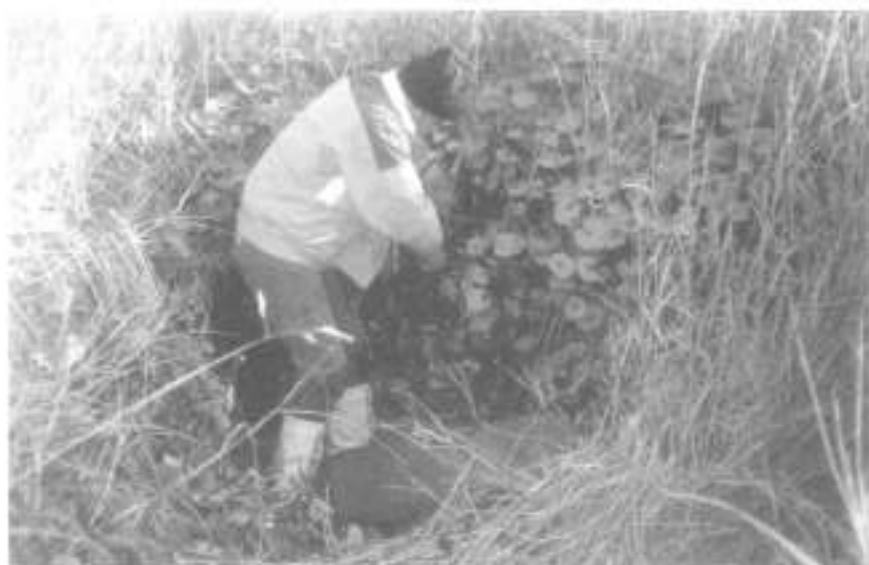
Carlos Dipilato working at the foundations of Luis Figue's house at Buen Suceso, near the outlet of the river at the southern end (April 1998).
