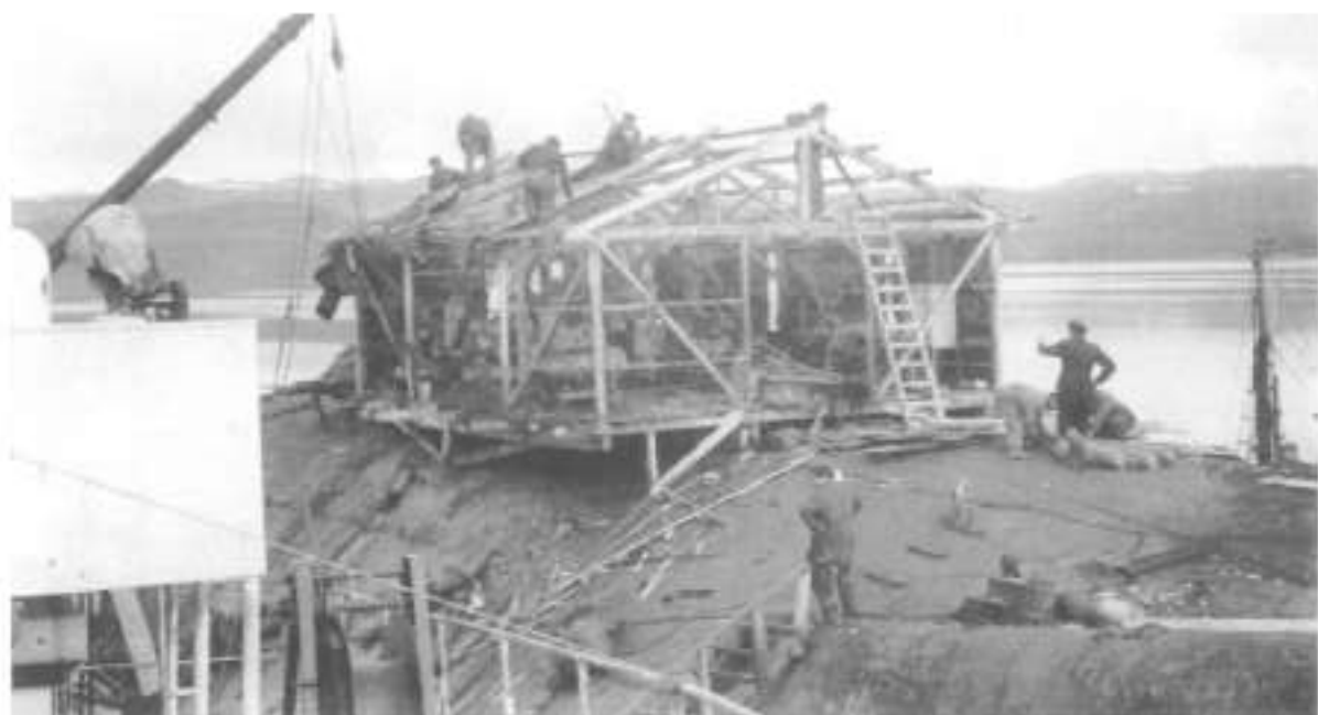
Dismantling the small shed used by divers and operators during the attempt to rescue the ship (1954).
