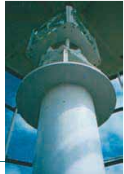
The optics of San Antonio Lighthouse and details of the emergency gas lantern powered with 900 candela.
