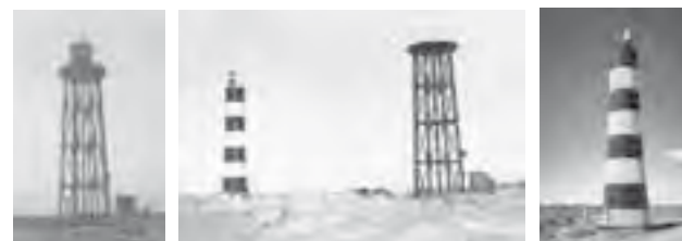
Images taken of the old iron truncated pyramid tower, which was later replaced by a cylindrical tower.
