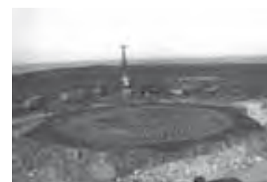
The beginning of the lighthouse construction: land conditioning.
