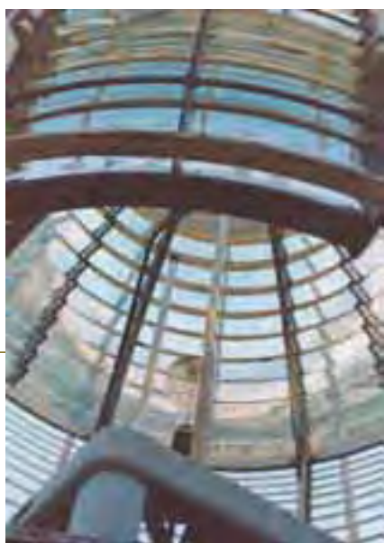
Details of the optics of Querandí Lighthouse, inside view.
